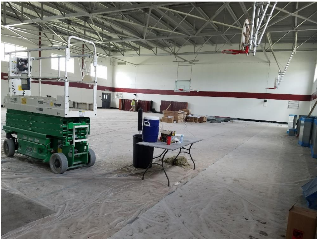
Figure 1 - Gymnasium Interior Demolition
