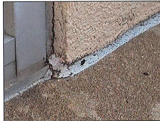
Exterior #7: Deteriorated Sealant at EIFS termination.
