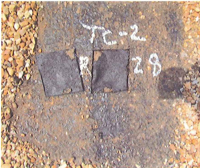
26. Test Cut #2 - Roof membrane removed to reveal perlite
