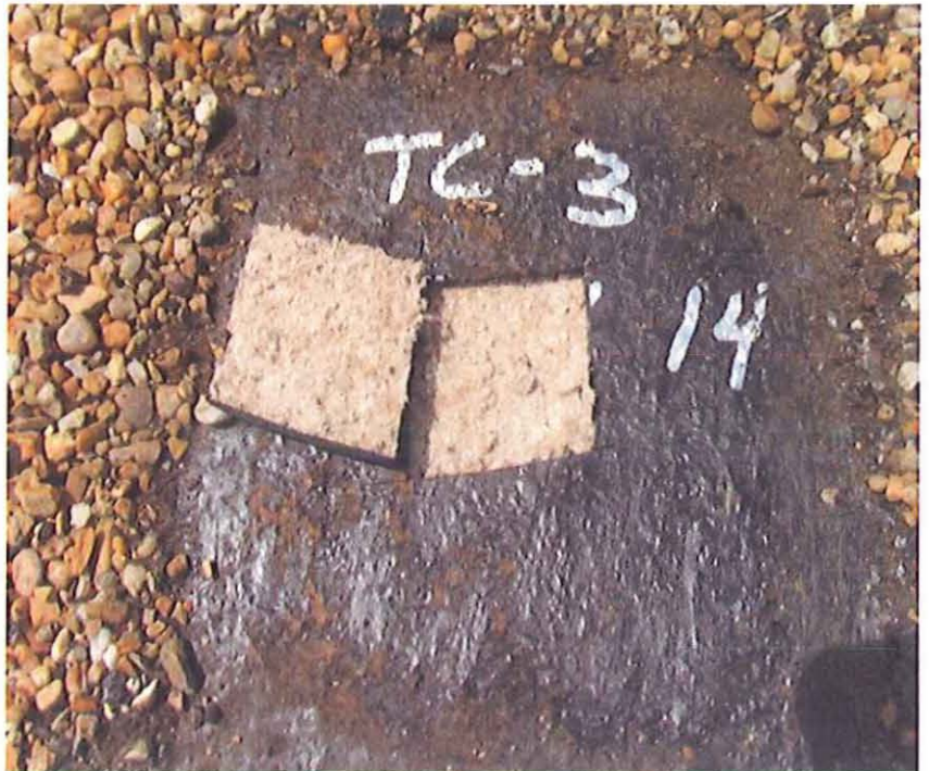
30. Test Cut #3 - Roof membrane removed to reveal perlite
