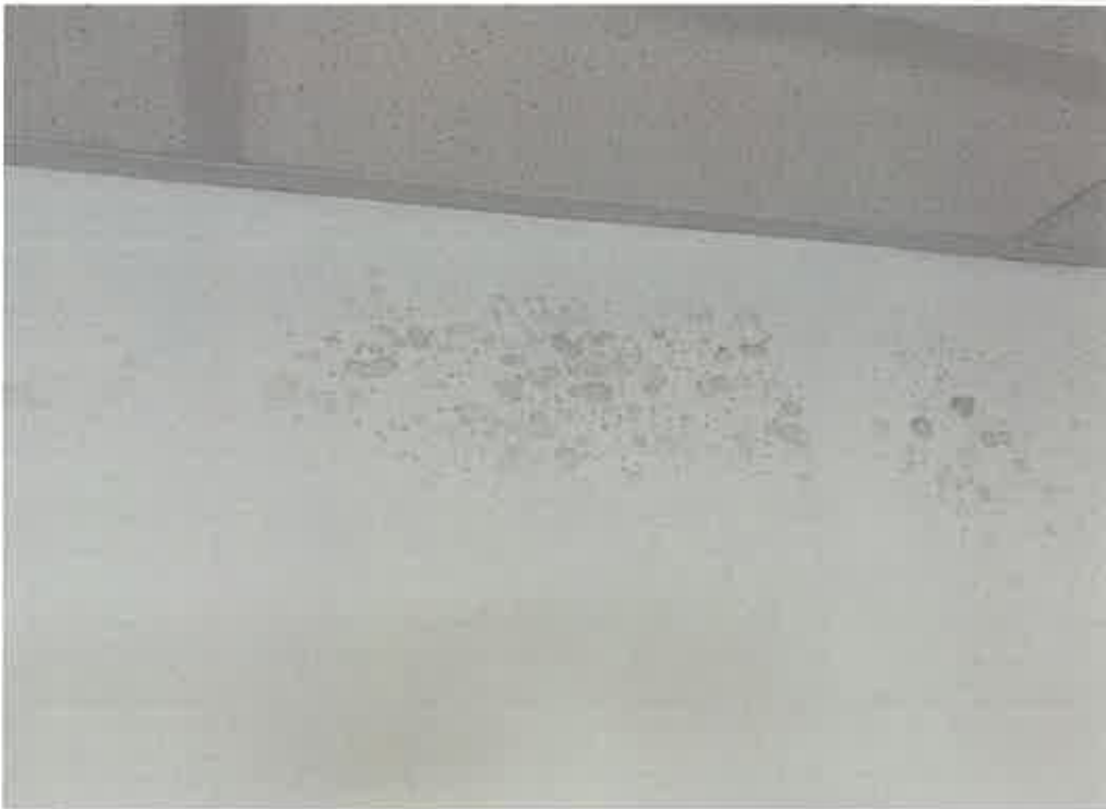
Photo 2: Meeting Room - Visible mold on the wallboard in the air flow path of the diffuses
