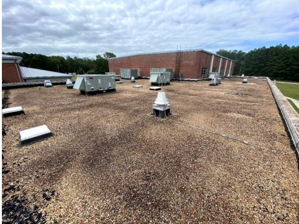
Photo 3: Southwest lower roof section.
