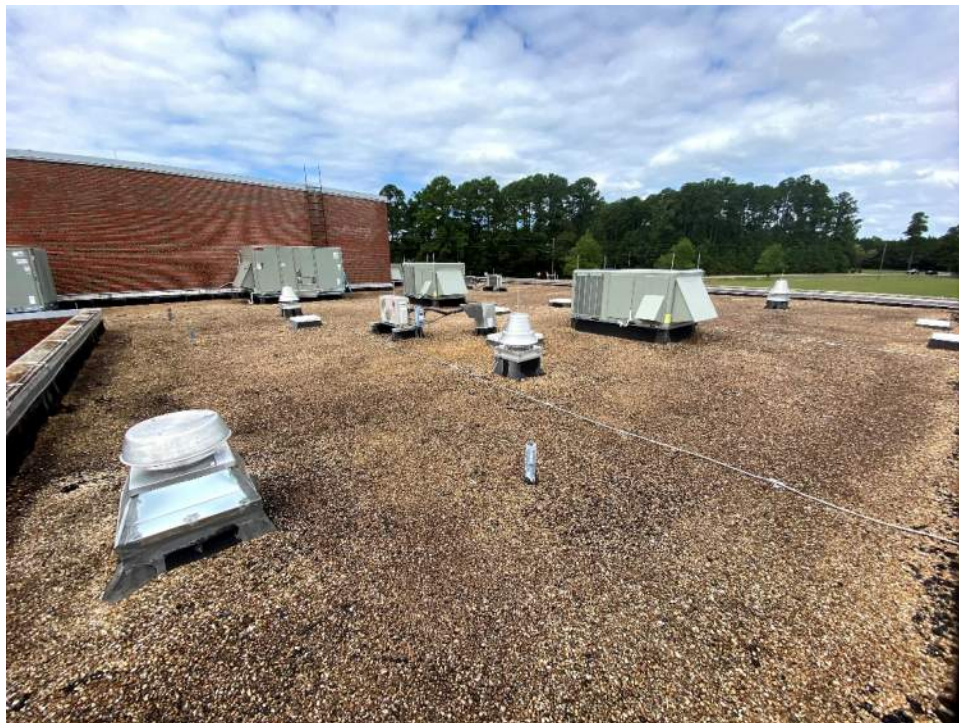
Photo 4: Northwest lower roof section.
