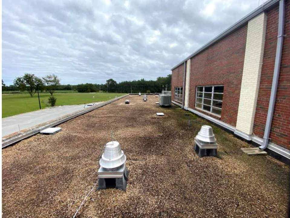
Photo 5: East lower roof section.
