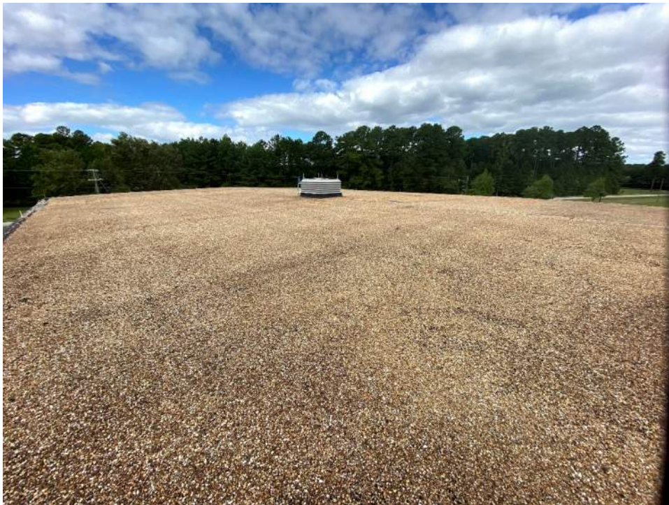
Photo 2: Northwest gymnasium roof section.
