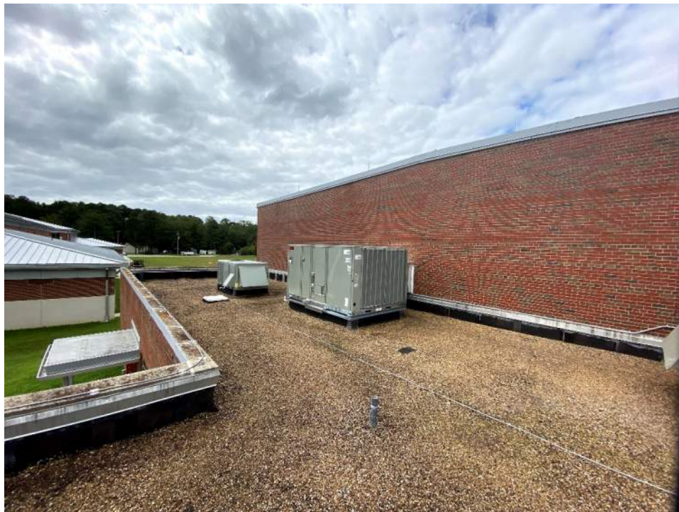
Photo 6: South lower roof section.
