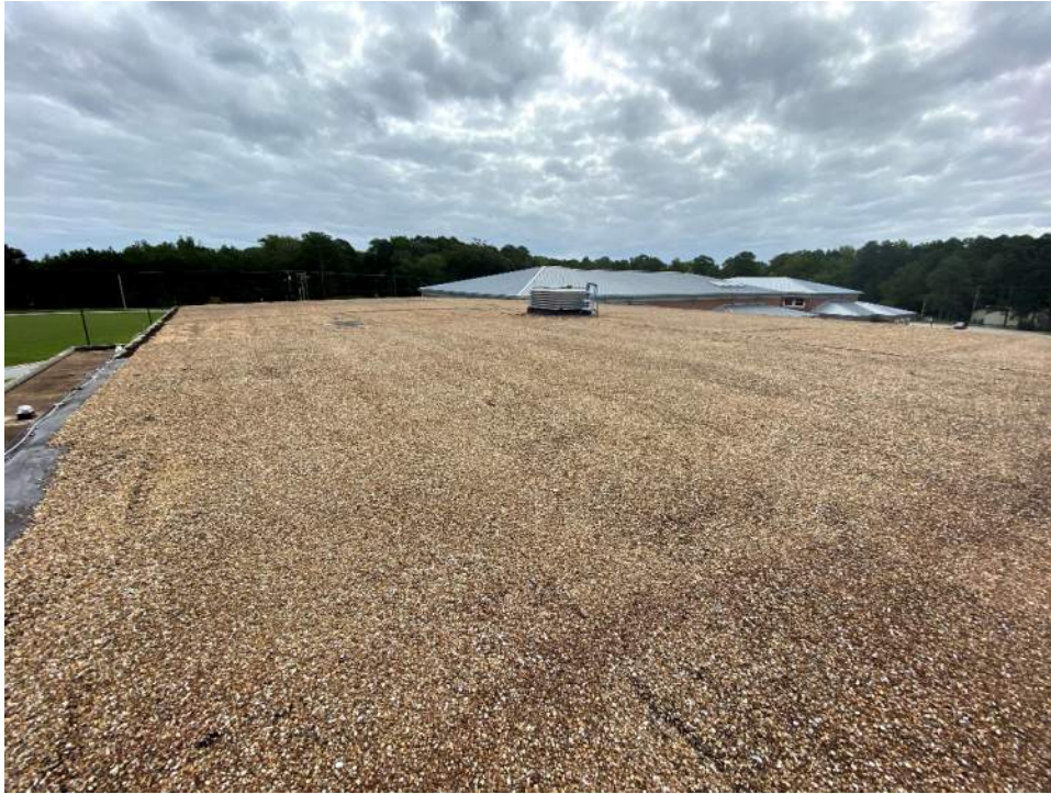
Photo 1: Southeast gymnasium roof section.
