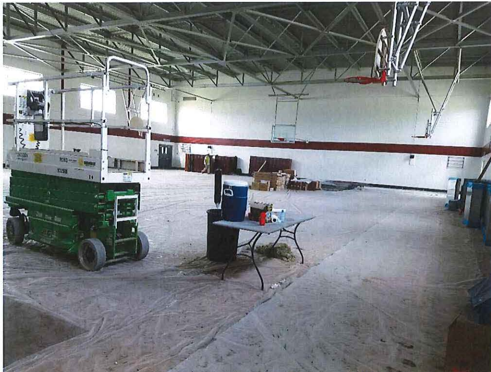
Figure 1 - Gymnasium Interior Demolition
